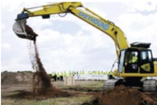
Transport Minister, David Jamison cuts the first sod.
