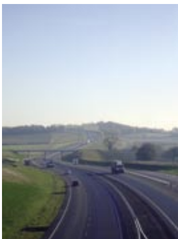
The finished bypass
