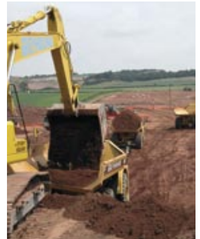
A38 tie in to Hints Hill
